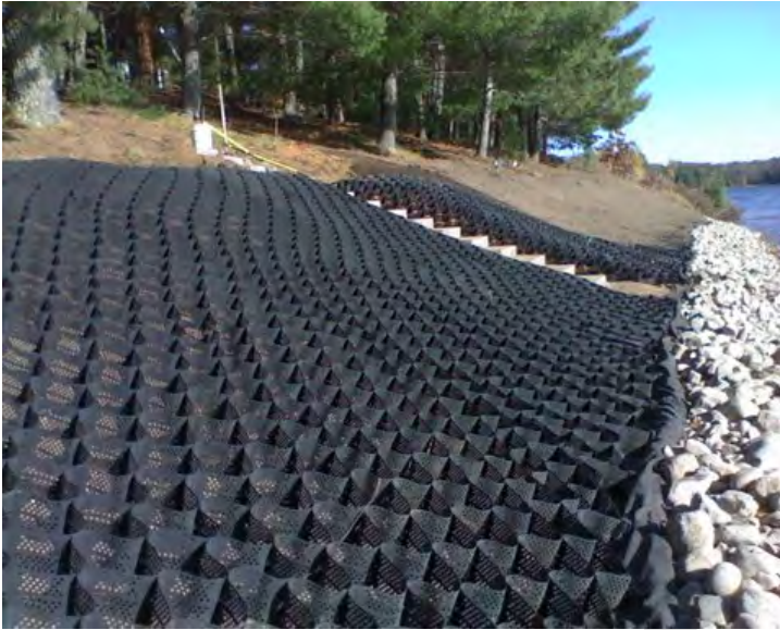
Photo 1. Geoweb cellular confinement structure. Photo courtesy of Menominee County.
